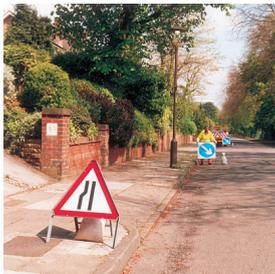
3. Using the appropriate diagrams in this Code to help you, work back towards the site, placing more signs as necessary. Keep on the verge or footway if you can. If you are on a two-way road, repeat this procedure and place signs for traffic going in the opposite direction, then cone off the works.
