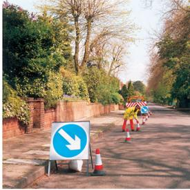
4. Always face the oncoming traffic when you set out the cones for the lead-in taper. Start from the kerb or road edge, working out towards the works. Complete the coning around the works, leaving enough room for working space and safety zones.
