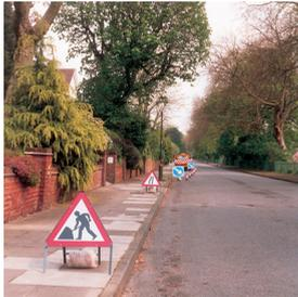
5. Use cones, 'Keep right' signs, barriers and road warning lights, and an information board to complete the warning, guidance and protection for the works.
