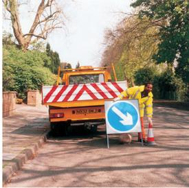
1. You must park your vehicle safely. You can park off the road in a position that does not obstruct a footway or cycle route. If you park in the road, you must protect it from traffic going past. Set up a 'Keep right' sign at the outside corner of the vehicle, along with a traffic cone.
