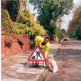
2. Set out the 'Road works ahead' sign. Measure or pace out the appropriate distance (D) from the point where your lead-in taper will begin. Then put one sign on the left-hand side (viewed from the perspective of traffic facing the sign) and another on the right-hand side of the road if your risk assessment deems it necessary. (Consult the table in the inside back cover of this Code for the appropriate distance D for different sites).
